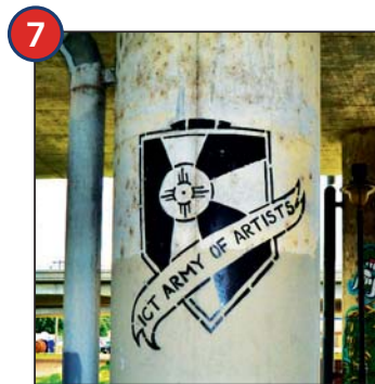
7 Douglas & I-135 Overpass Column
